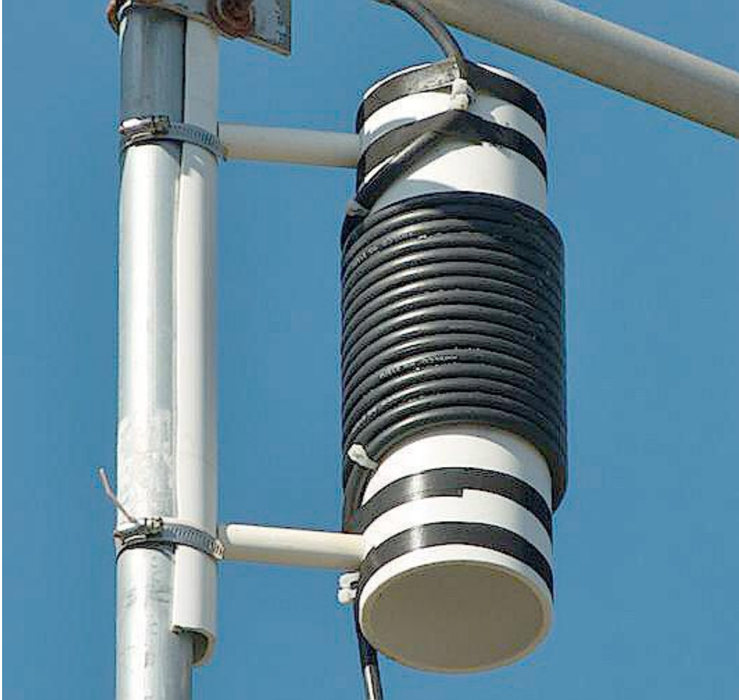
Update 04-2011....showing stainless steel clamps in final installation
