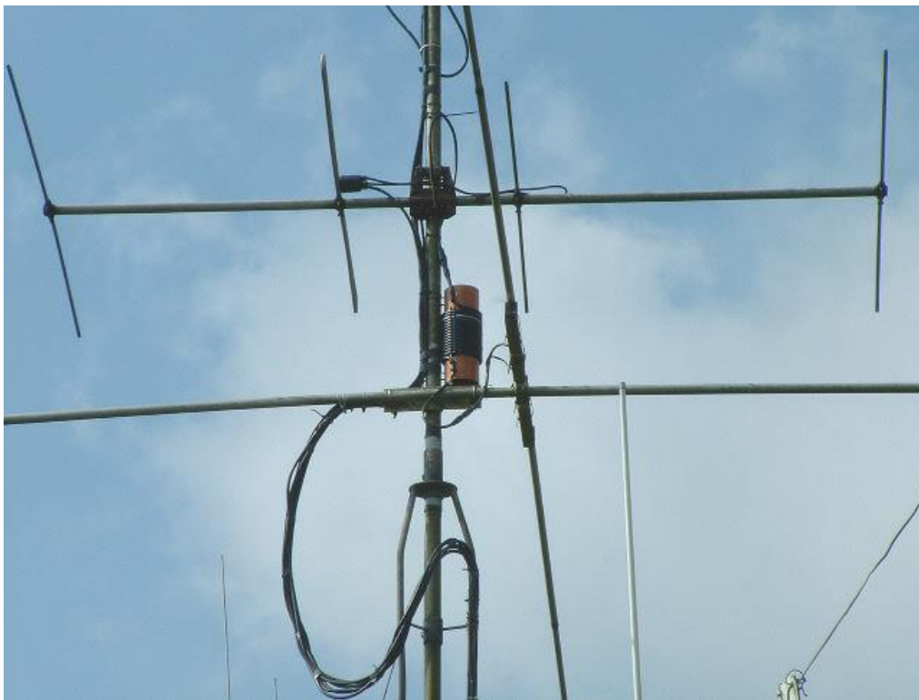
Courtesy of G4APL. (Air choke used on Mosley Mustang Mark3 3 element 10,15, 20 metre trapped Yagi)
